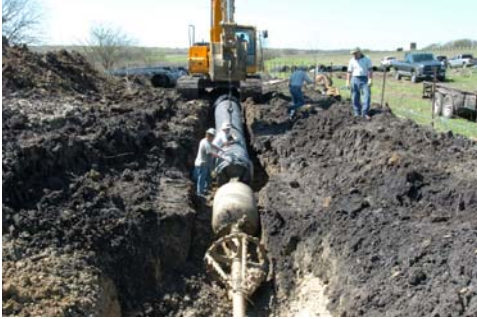
Figure No. 6 - Borepath Ramp
