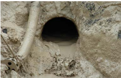
Figure No. 5 - Borepath Opening
