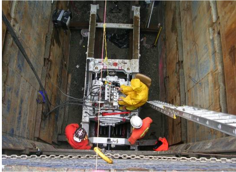
Figure 4: PT Unit and Jacking Frame
