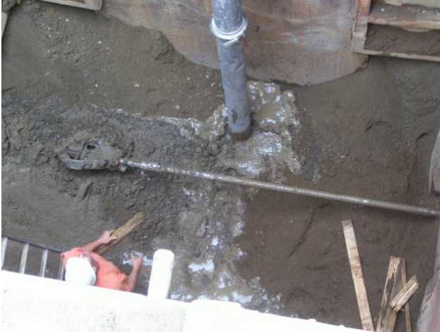
Figure 6: Reamer on HDD Rods
