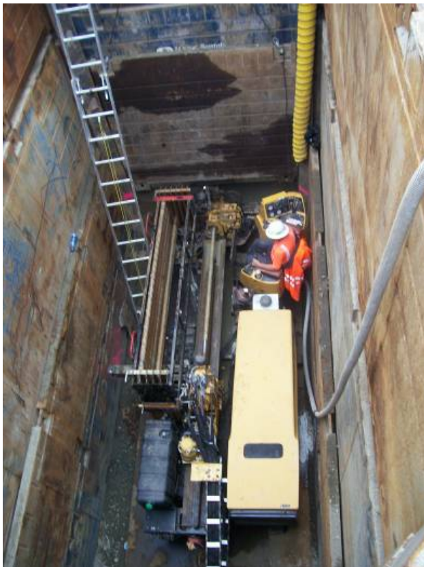
Figure 5: HDD Machine in Pit
