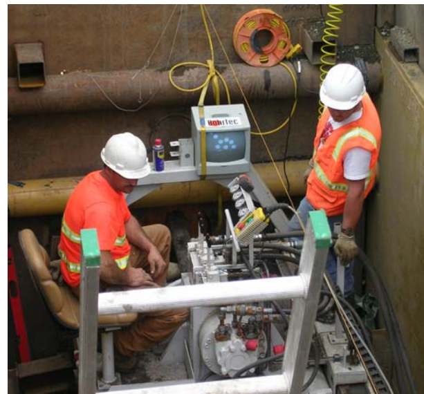
Figure 3: LCD Monitor in Jacking Pit
