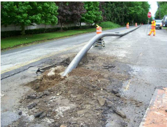
Figure 8: HDPE Pipe being pulled in
