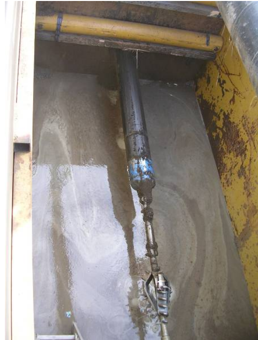
Figure 8: HDPE pull complete
