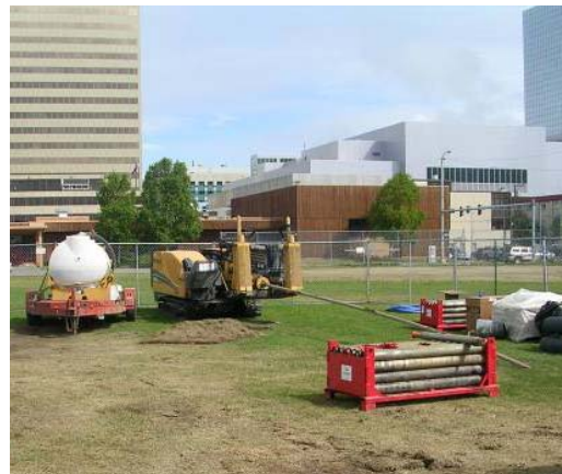
Figure 10: HDD rig pulling in pipe
