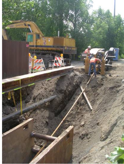
Figure 6: Sloped Path for Drill Rods
