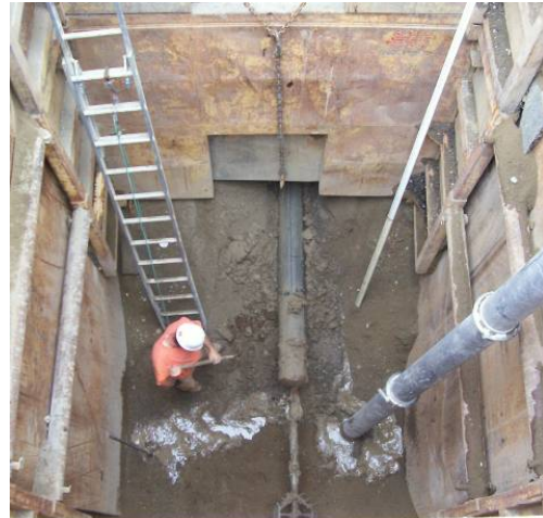
Figure 7: Reamer, Swivel and HDPE Pipe
