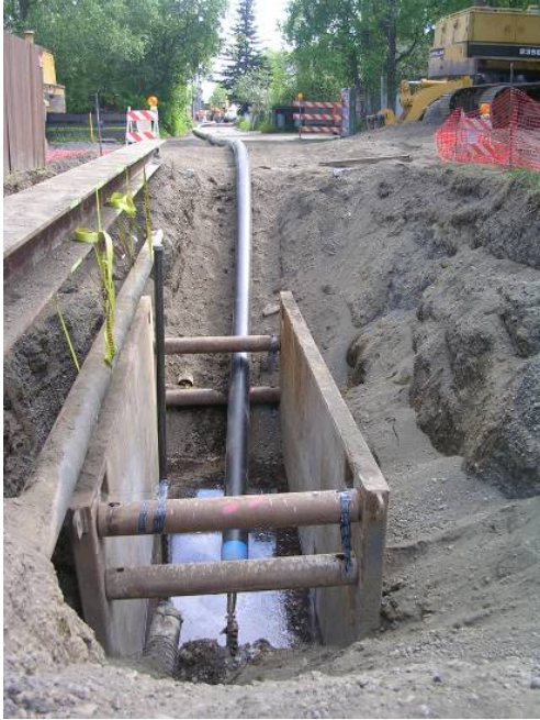
Figure 9: HDPE pipe being pulled into the bore
