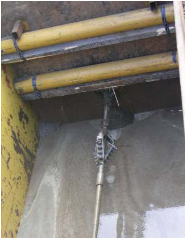
Figure 7: Shredder Reamer
